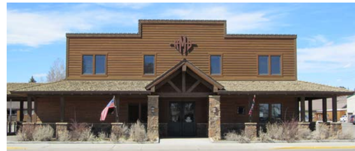
Combination of stepped parapet and open timber gable.
