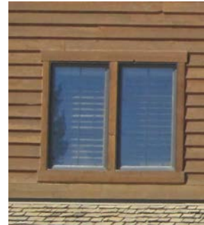
Appropriate window detailing.
