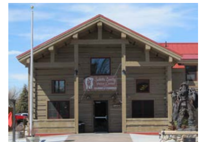
Open gable with heavy timbers.
